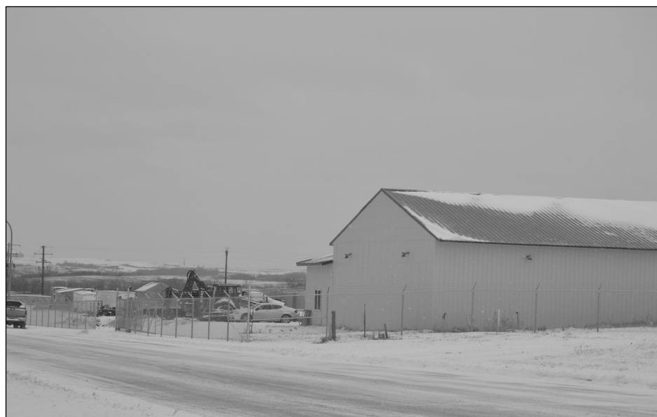
The back of the hall is all fenced up so one has to go through the fence in order to get in the back of the hall.
