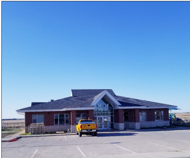
New Headstart building that has been waiting all year for the high school to be completed so they can move in their building. The move is scheduled for Fall.
