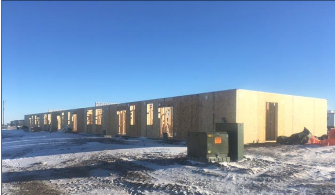
Apartment picture shows most of the outside work completed.
