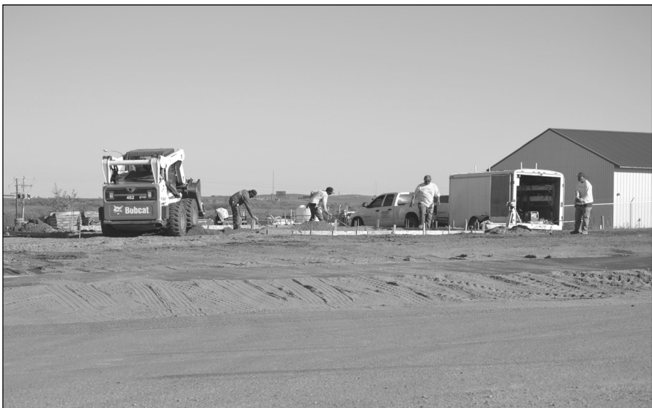
Here is another angle of them working on the wall.
