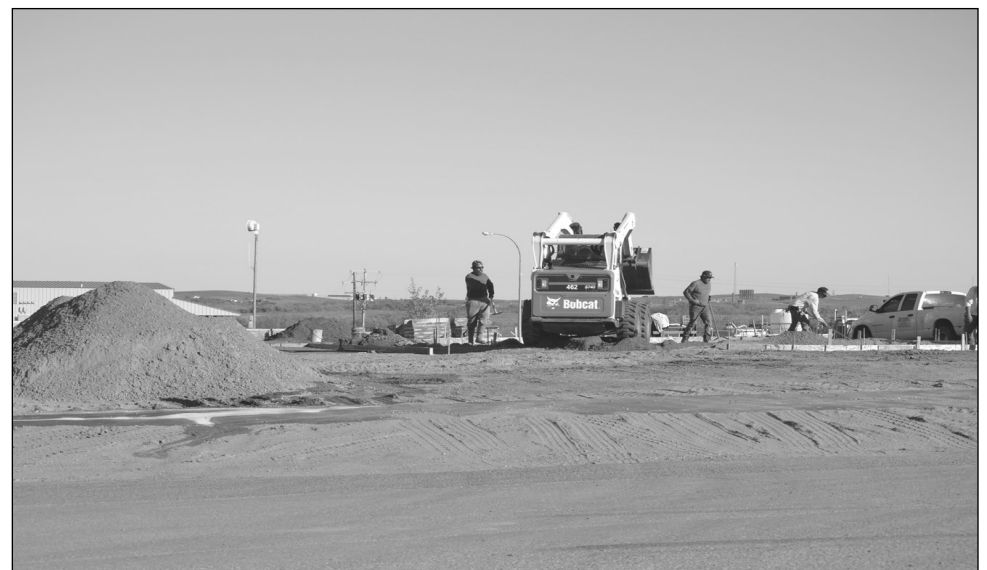
Front side of these guys working on the Veterans Wall.
