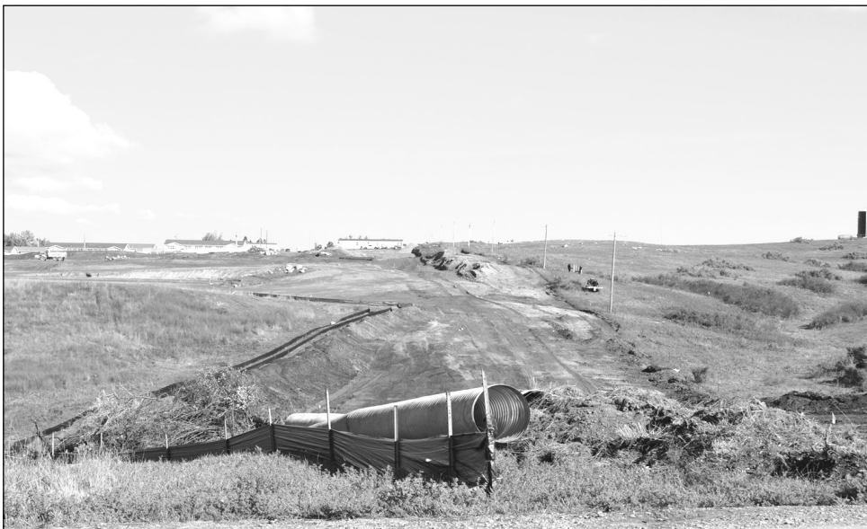
These culverts have yet to be put in place which are probably already in place since this picture was taken.
