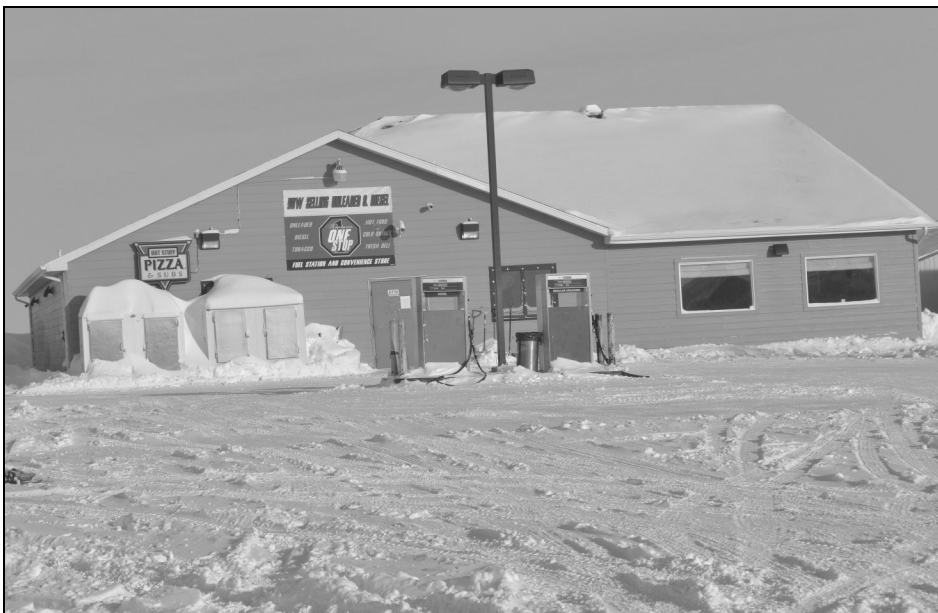
Mandaree One Stop was surrounded by piles of snow.
